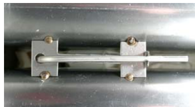
Typical high-limit/sensor probe locations and mounting hardware.
